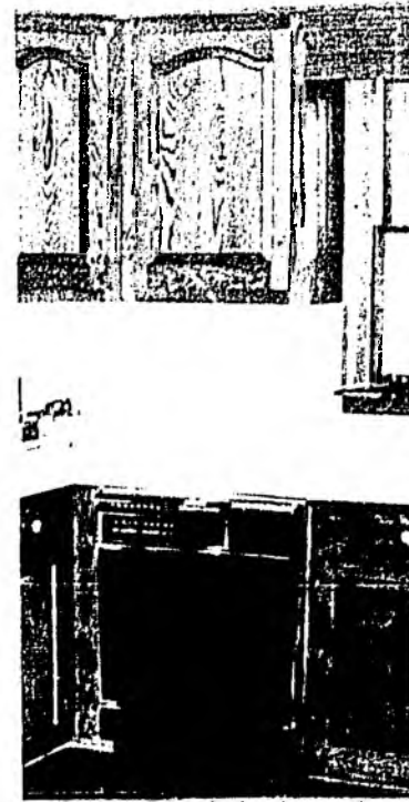
(Top) This photo shows the arch that is formed by bending the wood on a form; (left) a set of cabinets that was one of the first projects that the two men undertook; (left) this mantle was built from a picture that the customer liked.
