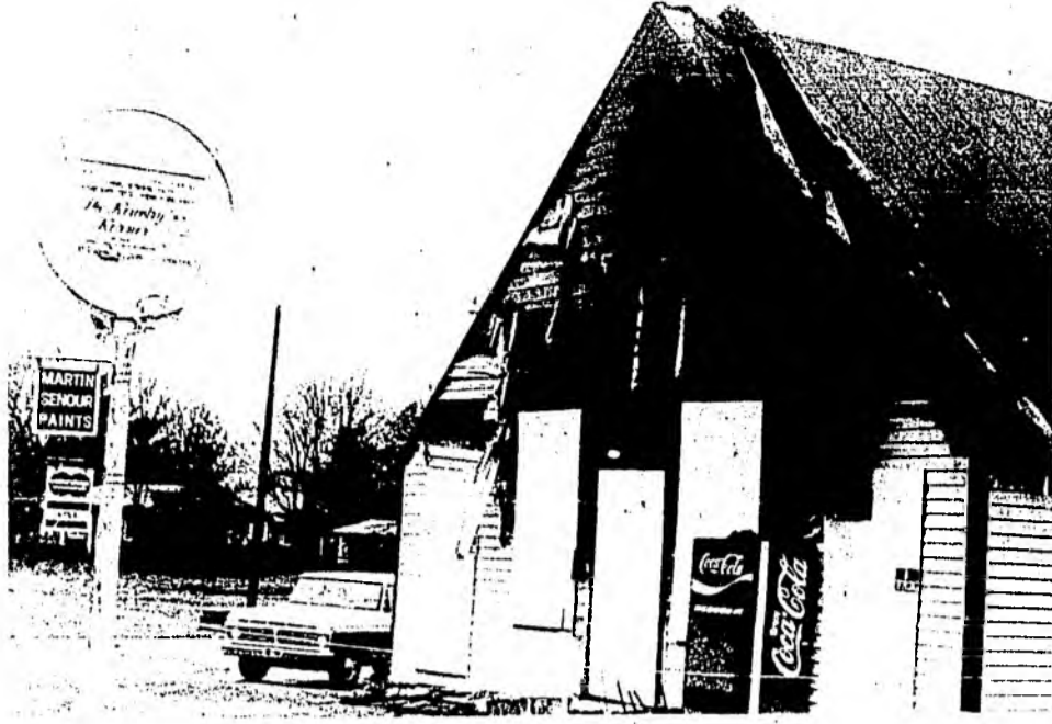
An electrical malfunction has been cited as the possible cause of a Thursday morning fire which gutted the Kountry Korner.
