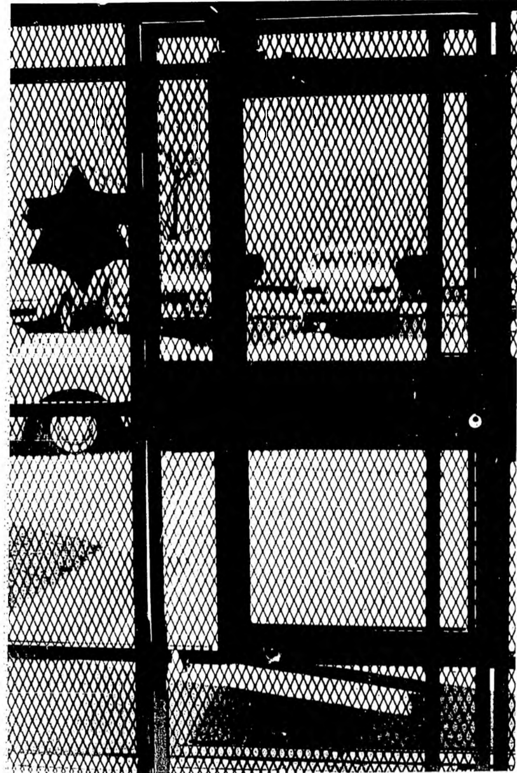
Installed about a month ago, the County Jail's newest security measure is a metal grate which stretches across the jail's front entrance. (Photo by John Vernelson)
