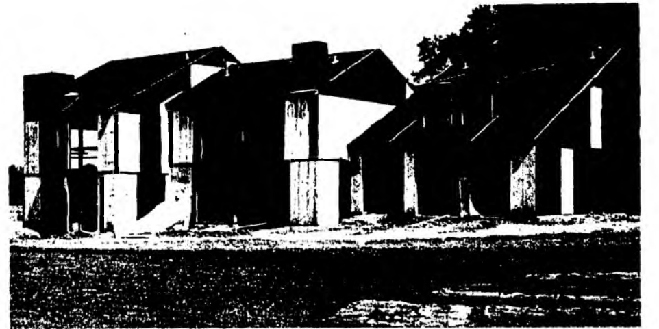
More Golfdominiums under construction by Salem Ventures.
