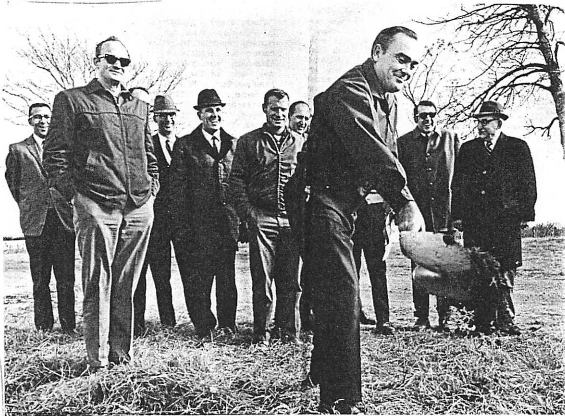
Chairman of the Davie Board of Commissioners, John M. Bailey is shown above breaking the ground at the site of the new club house for the Hickory Hill Golf and Country Club while members of the board of directors and visitors watch.
