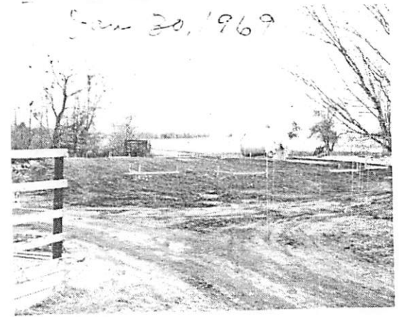
..... Site cleared for Hickory Hill Club House.
