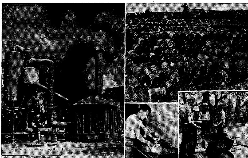
How empty oil drums are being used in the Pacific area is shown by these photos. Left, the drums were used in asphalt plant, as stacks, etc. Center, household use, wash sinks made from drums. Upper right, view of one of the oil drum farms. Lower right, used for barbecue. Other uses include bomb shelters, gateway arches, legs for water tanks, incinerators, sewer pipes and reflectors on light poles.
