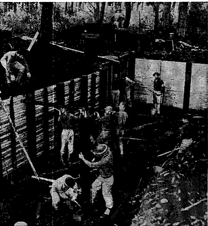
U. S. troops and native workmen work on underground installations of dugouts. This is a first aid dugout equipped to perform surgery in an advanced position.
