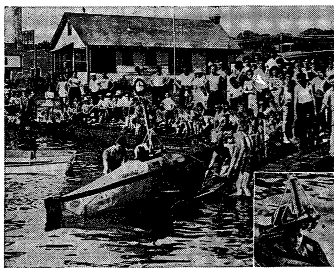
Barney Connett of Chicago, master and crew of an 11-foot submarine, previous to making a successful test dive in the salt water of the Hudson river in Yonkers, N. Y. Connett, in his homemade sub, has made approximately 400 dives, once crossing Lake Michigan under water from Chicago to Michigan City, Ind., a distance of 37 miles. The sub is powered by two sets of batteries and has all the usual submarine equipment.
