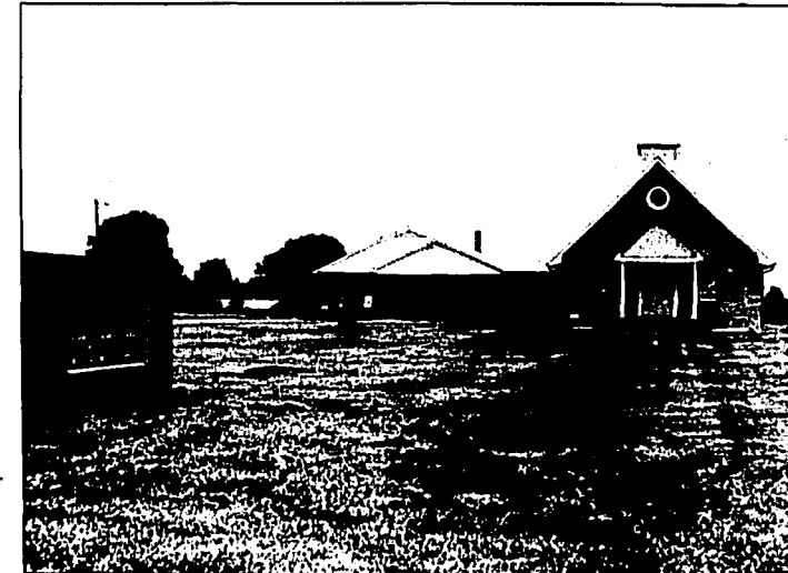
Cornatzer United Methodist Church as it looks today, located on Cornatzer Road.
