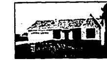
TWINBROOK -Brand new home just waiting for you. 3BR/2BA Energy efficient with vaulted ceiling in living room. Cherry cabinets throughout. $93,500.00
