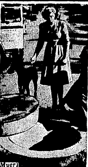
WOOD SUBSTITUTE —Los Angeles engineer built wooden manhole covers out of timbers treated to resist termites and decay when shortages threatened to delay sewage construction.
